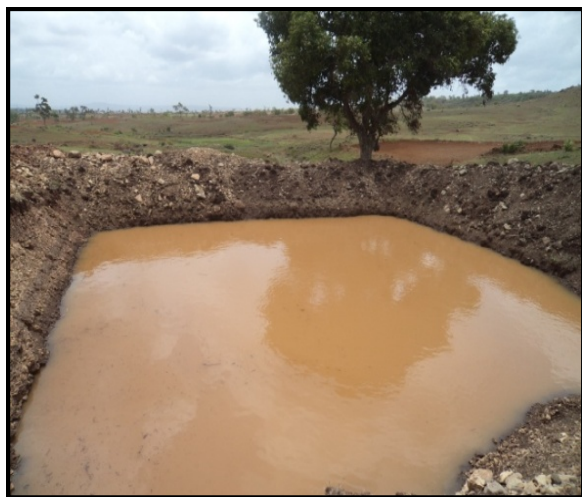
Figure 4. Farm pond immediately after construction
